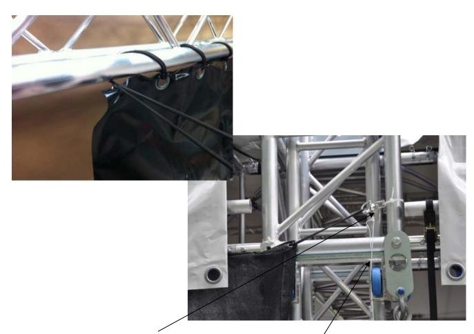
The quick release hook has to fixed with a plastic retainer on in another way.
