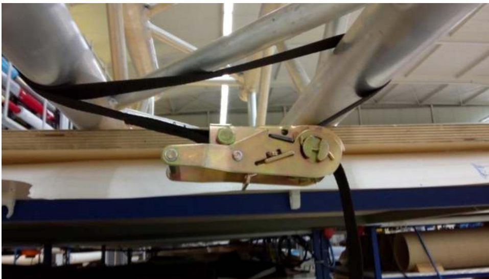
Placing the ratchet under the truss
